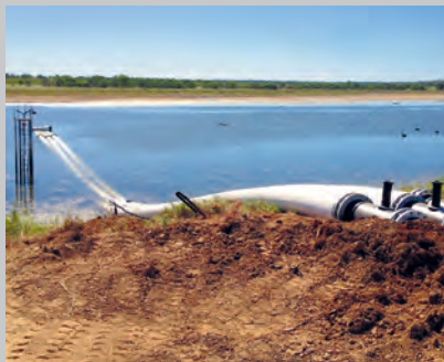
Crinum Siphon Project - Install of 450mm Poly Pipe
