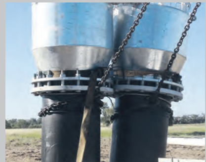
Crinum Siphon Project - Install of 450mm Poly Pipe
