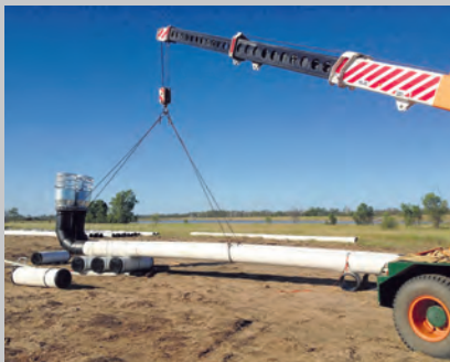
Crinum Siphon Project - Install of 450mm Poly Pipe
